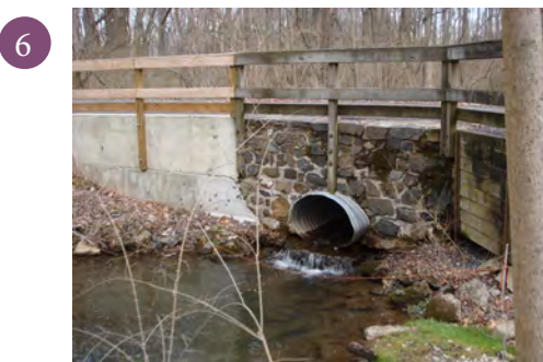
Culvert - This culvert concentrates the stormwater flow and increases erosion.
