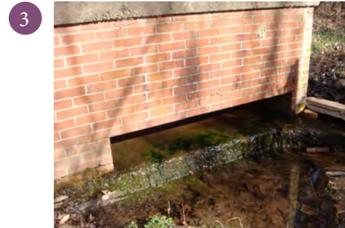
Stormwater Outfalls - Stormwater from the neighborhoods are piped directly into the creek.
