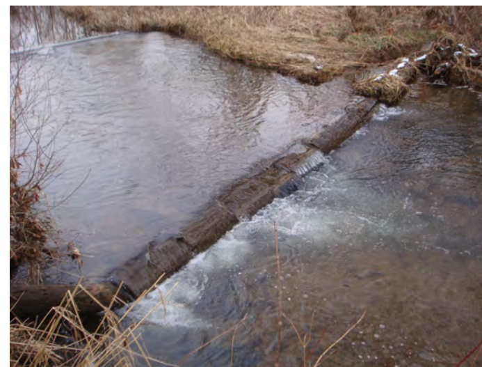
Figure 38: Creek sill design by John Munro of Munro Ecological Services installed at Pennsburg Nature Preserve.
