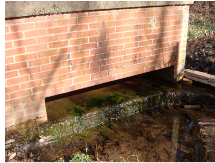
Figure 14: Brick headwall stormwater outfall.
