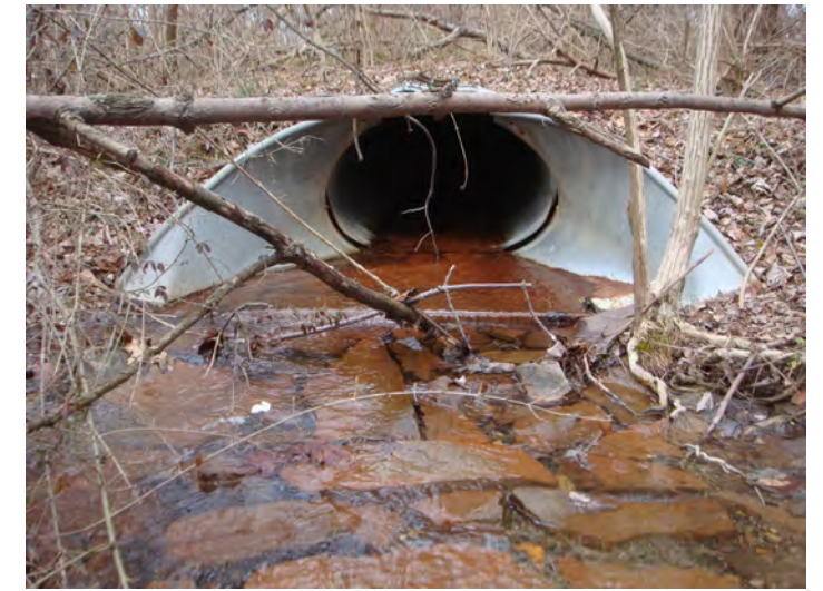
Figure 15: Second stormwater outfall.
