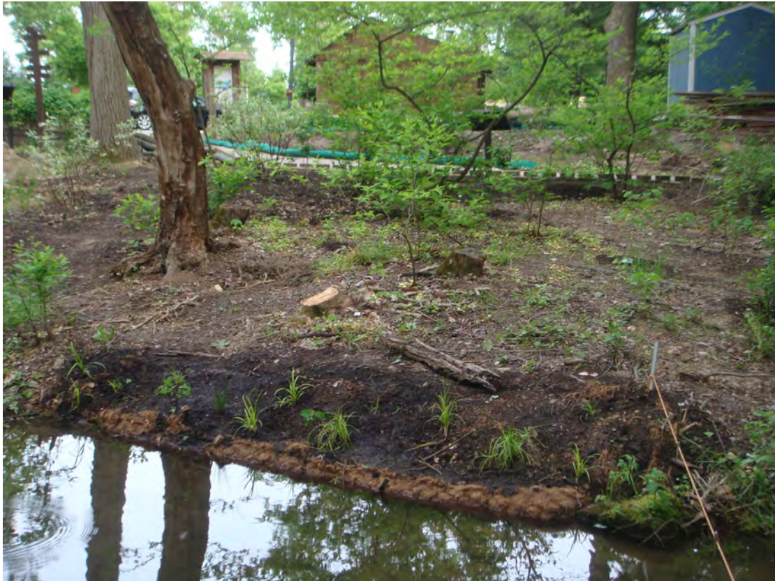
After - Closeup view of streambank stabilization
