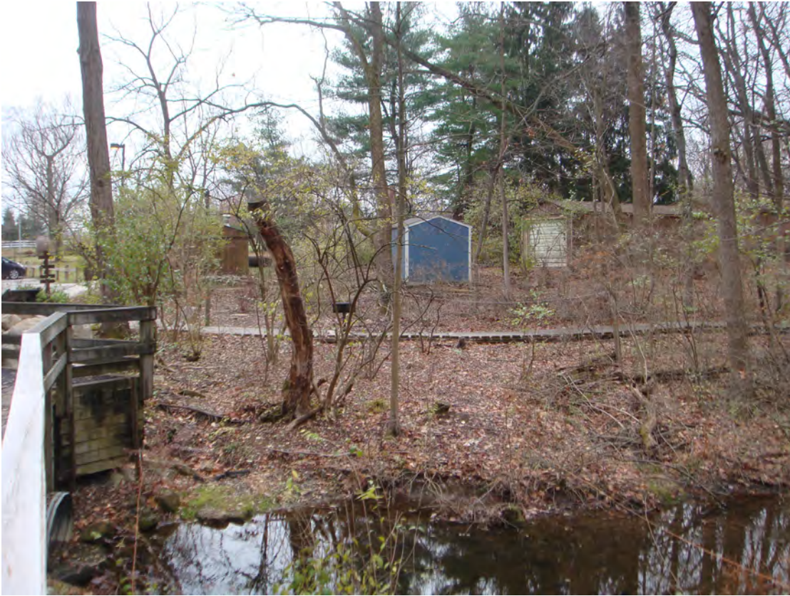
Before - Two eroded stormwater channels (right and left sides) and eroded streambank (middle). Also many exotic plants (bush honey suckle and privet).
